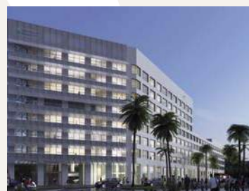
CONNEXIO (BNP Paribas Real Estate/UNOFI) Business offices (11 000 sqm)
