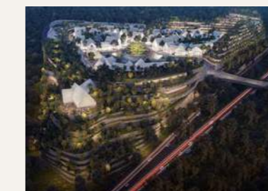
VILLAGE DE SOPHIA (Cie de Phalsbourg) 75 000 sqm mixed-use development: hotel, retail, services and business offices (20 000 sqm)
